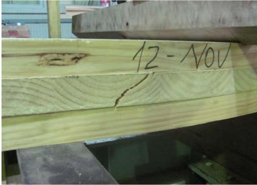
Figure 1: Typical rolling shear failure in a CLT plate subject to bending
