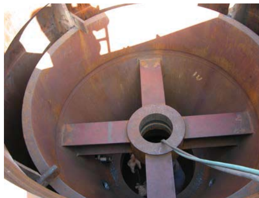
Figure 6. Picture of cross support structure
