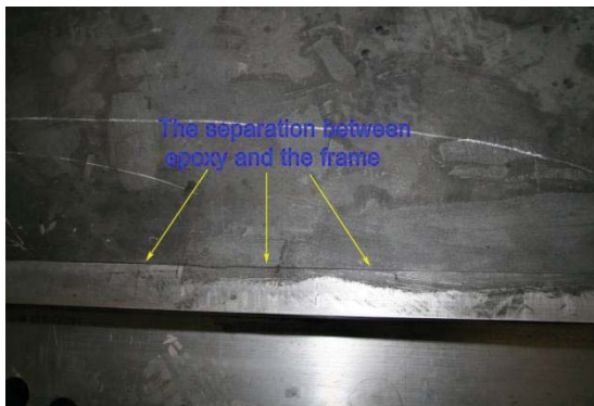
Figure 3. The separation between epoxy resin and the frame of nozzle
