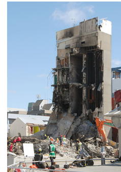
Fig.2 Remains of the building after the earthquake [2]
