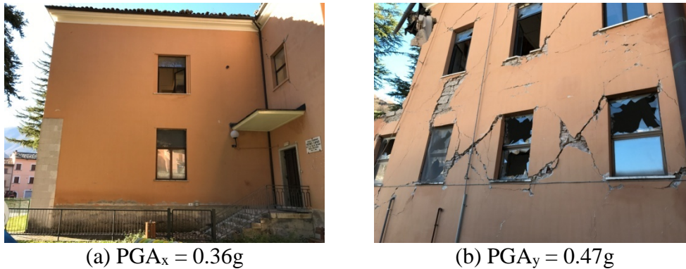
Figure 12 - Comparison between the damage distribution obtained in the walls oriented in X (a) and Y (b) after the Mw 5.9 earthquake of October 26 th .
